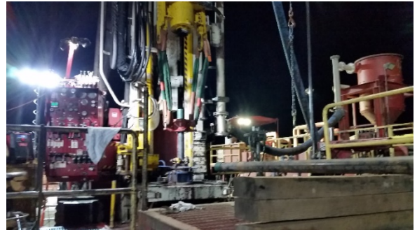
Clear Creek used a simple analytical model and aquifer testing results to demonstrate sufficient on-site groundwater resources for the project.
