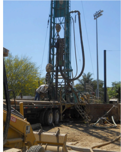
Drilling on campus at CBU
